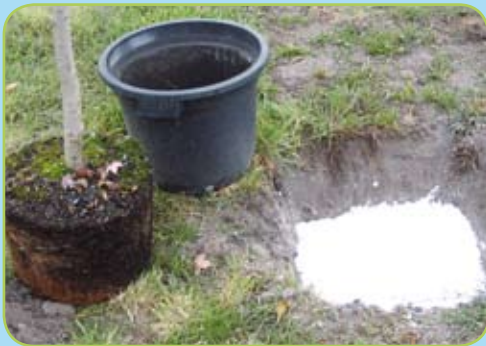
Hydrocell placed in the planter hole ready for a 45L root ball.
