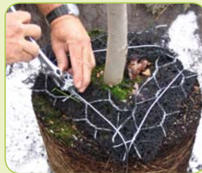
Street tree stable and secure, using the Platipus anchor system.
