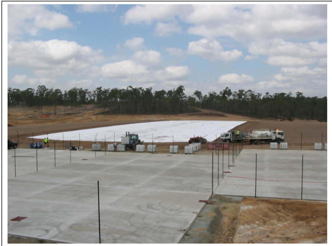
Fytofoam layer application in October 2005.
